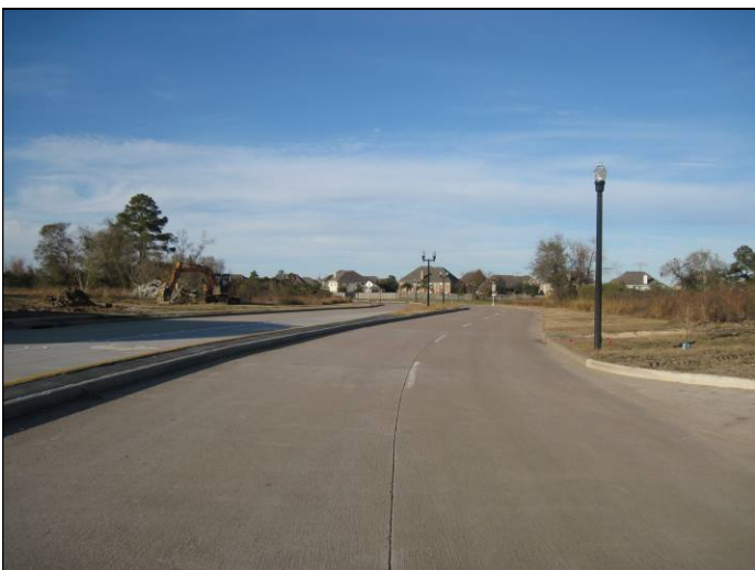
VIEW OF LAKESIDE DRIVE
