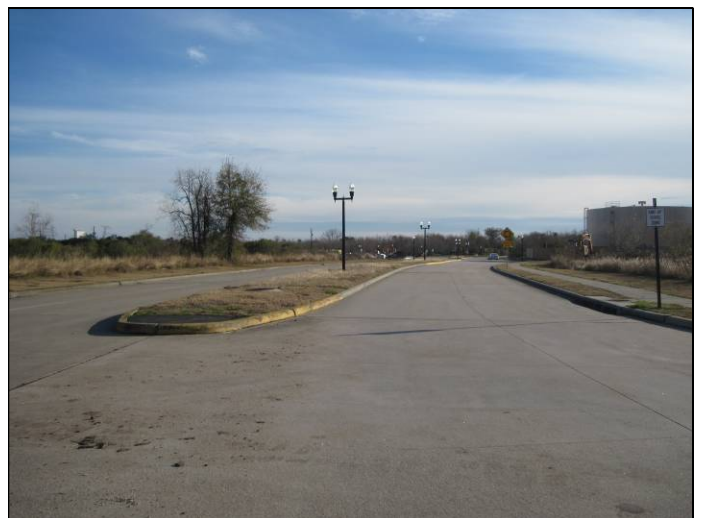
VIEW OF LAKESIDE DRIVE
