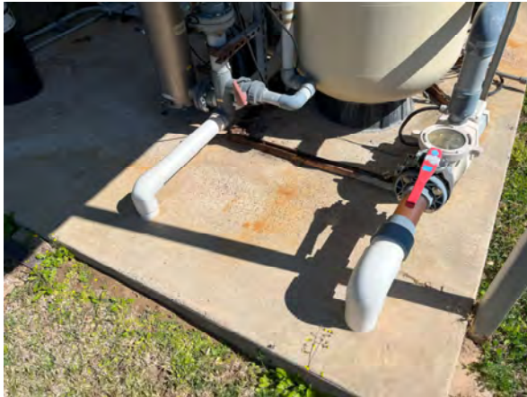
Photo #7 View of Splashpad slab floor penetrations.
