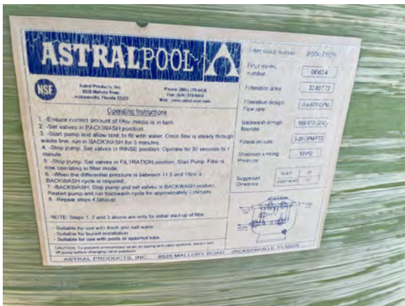
Photo #47 View of pool filter engineering specifications.
