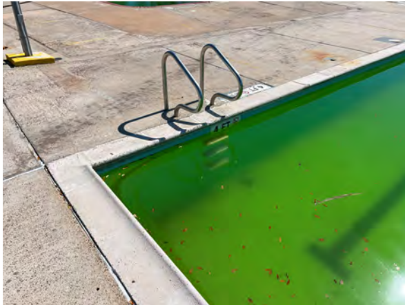
Photo #31 Example view of Lap Pool grab rail.
