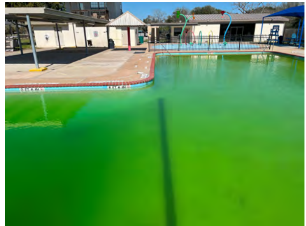
Photo #22 View of contrasting tile floor marking indicating change in floor slope in the Children's Pool.
