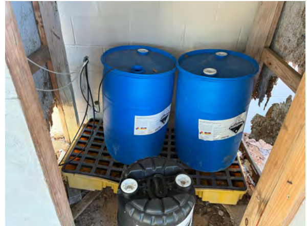
Photo #56 View of muriatic acid carboys on secondary containment platform.
