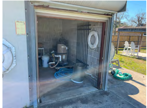
Photo #38 View of pool equipment storage and chemical feed pump enclosure with garage door open.
