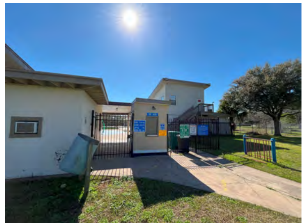
Photo #66 View of front entrance and access booth.
