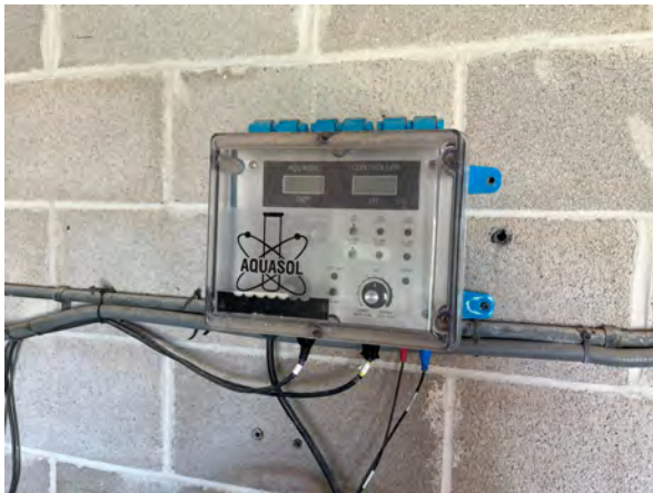
Photo #57 View of pool water chemistry controller.
