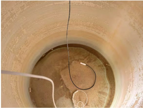
Photo #61 View of sodium-hypochlorite storage tank interior.
