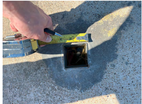
Photo #34 Example view of Lap Pool starting block anchor.
