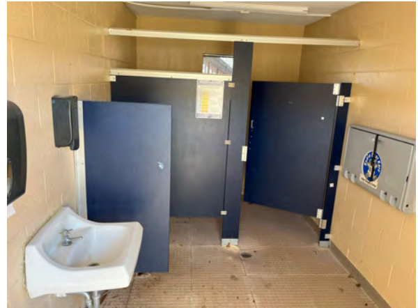
Photo #68 View of men's bathroom.
