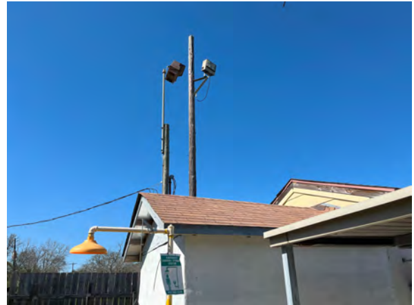
Photo #44 View of pool equipment storage enclosure roof and overhead lighting.
