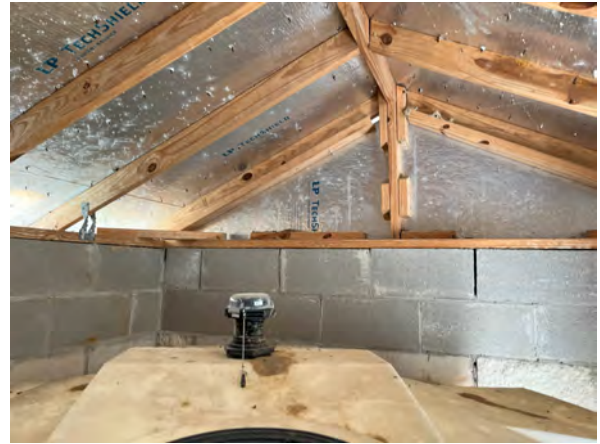
Photo #62 View of sodium-hypochlorite storage closet, above the chemical container.
