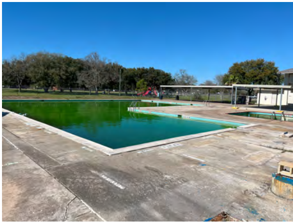
Photo #63 View of pool deck where Lap Pool waterslide has been removed. Concrete footings still remain.
