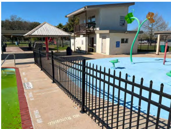
Photo #65 View of fence dividing the Splashpad area from the Children's Pool.
