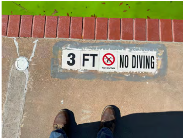
Photo #25 Example view of Children's Pool depth marking and "No Diving" signage.
