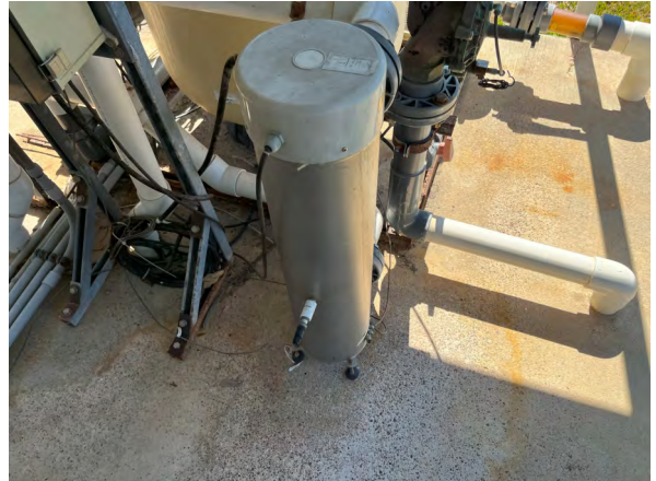
Photo #14 View of Splashpad secondary disinfectant UV system.
