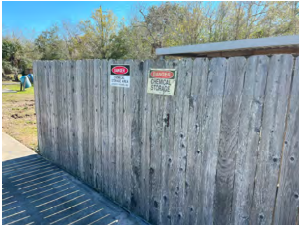
Photo #37 View of fence surrounding outdoor pool mechanical and chemical storage area.
