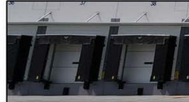
#3 INSULATED OVERHEAD DOORS WITH DOCK SHELTERS
