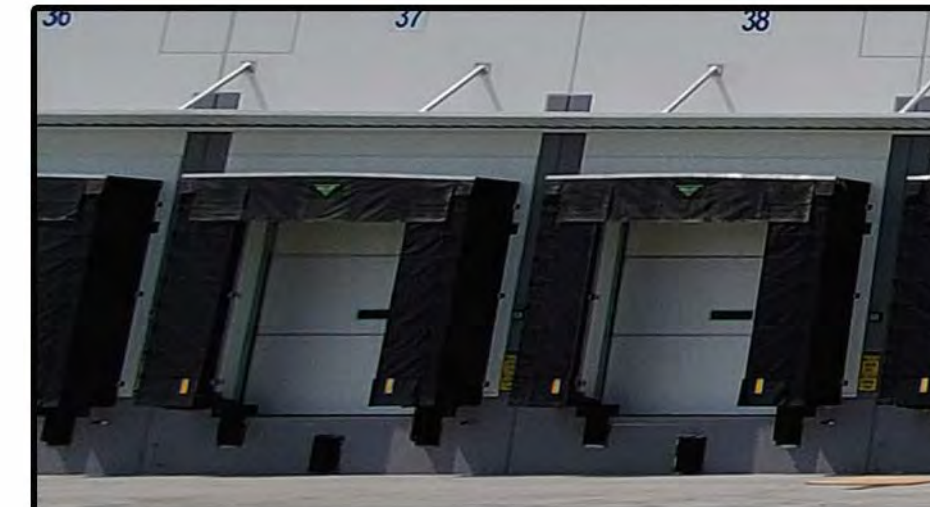
#3 INSULATED OVERHEAD DOORS WITH DOCK SHELTERS
