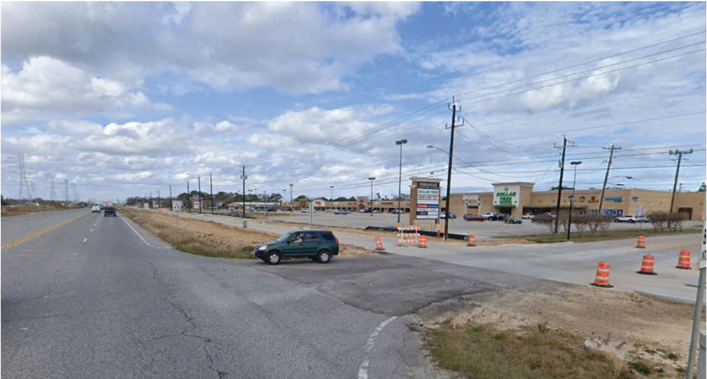
SH 146 (looking north)
